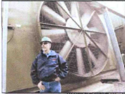
NANCY RICHMOND / Herald Jeff Spittler, BP's Durango operations manager, stands near the cooling fan for one of the four gas-fired compressors at the Dry Creek Compressor Station. The V12 engines produce 1,200 horsepower each, and are used to increase gas pipeline pressure from 50 pounds to 350 pounds and remove some water from gas piped in from about 100 surrounding wells.
